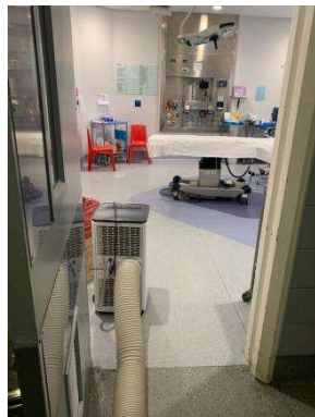
Figure 2: portable air conditioning unit in the operating theatre.
